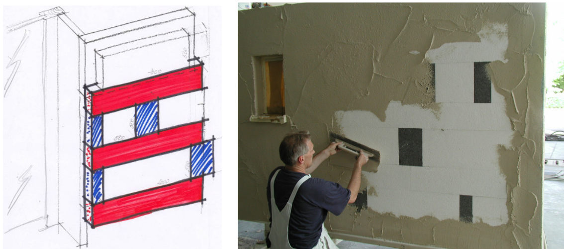
Figure 1: Schematical view of LockPlate®-System covering a wall using different baseplates and components (red=horizontal lock plate; blue= vertical lock plate) and production of the EOTA test wall
