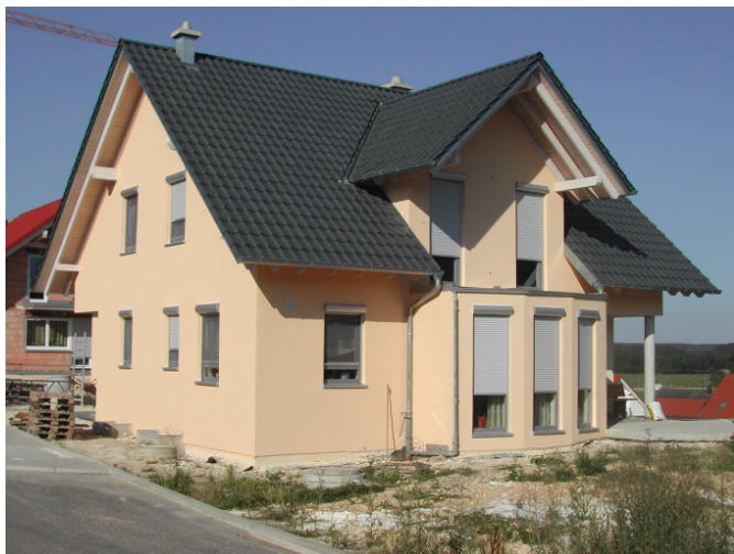
Figure 2: VIP-ETICS-facades of demonstration house Giengen/Burgberg
