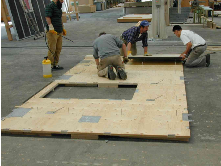
Figure 2: Prefabrication of the insulation elements
